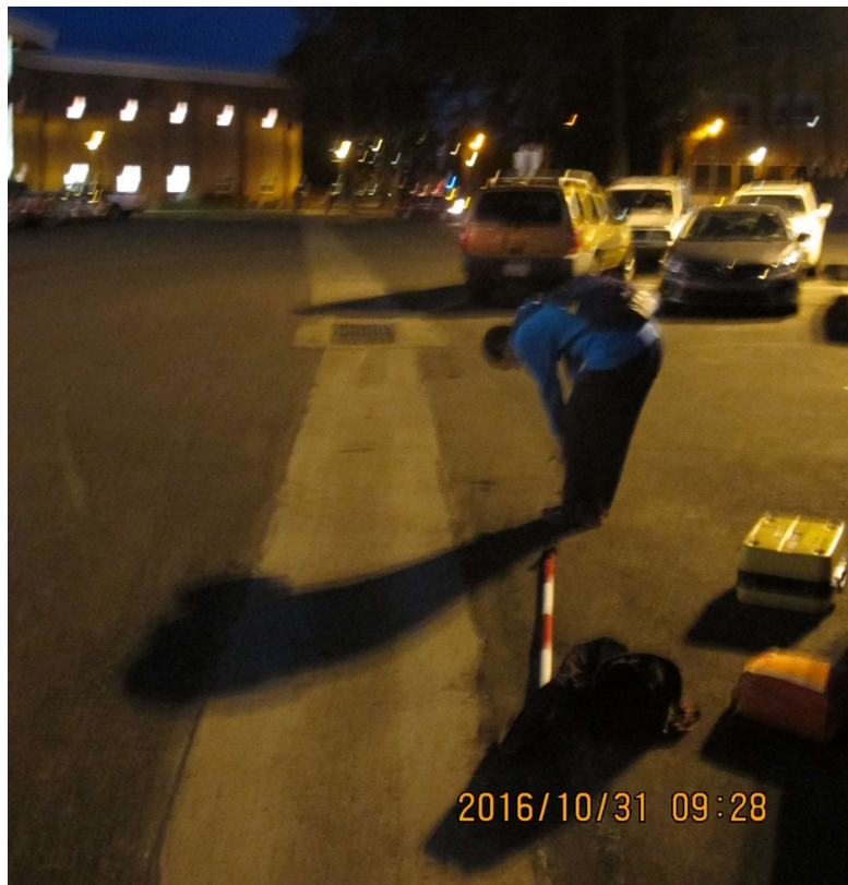
Figure 9: Current Storm Drain at Cline Library/Eastburn Education Watershed
